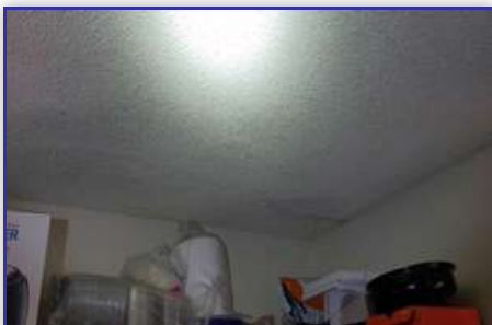
Location: 2ND FLOOR UNIT 1749/LIVINGROOM 4.2 Microbial growth /roof water stains
