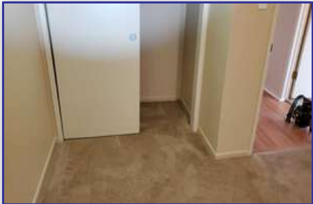
Location: 2ND FLOOR UNIT 1747 /BEDROOMS 3.1 Missing lower guides
