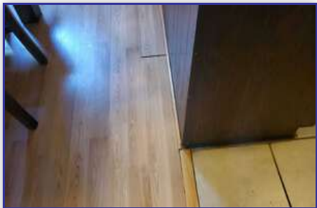
Location: UNIT 1745/ DINNING AREA 1.1 Poor flooring installation
