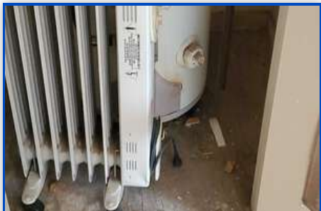
Location: 2ND FLOOR UNIT 1747 /WATER HEATER 3.1 Scorched marks
