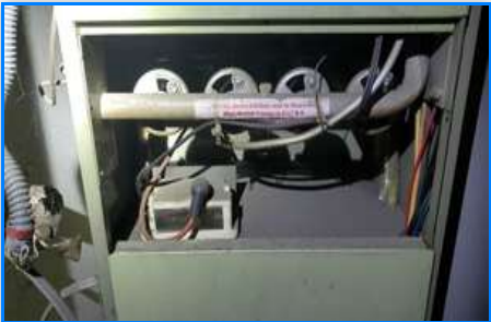
Location: 1745/ FURNACE 4.1 Service and certify unit (past life expectancy)
