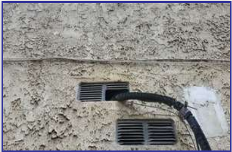
Location: EXT BUILDING 1.1 Damaged vents cover
