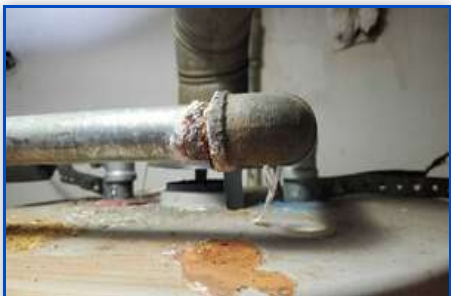
Location: 1745 WATER HEATER/GARAGE 3.1 Corroded galvanized water lines
