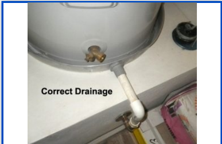
2.1 Water heater drip pan exampe
