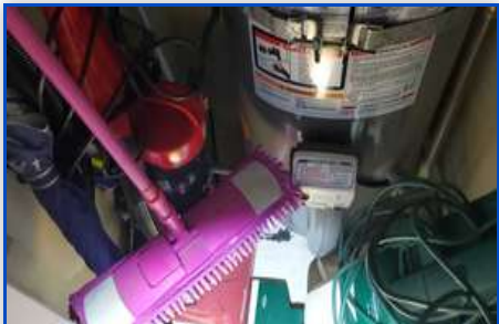
Location: 2ND FLOOR UNIT 1749/WATER HEATER 1.1 No drip leg
