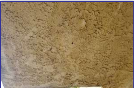
Location: EXT BUILDING 1.1 Typical stucco cracks
