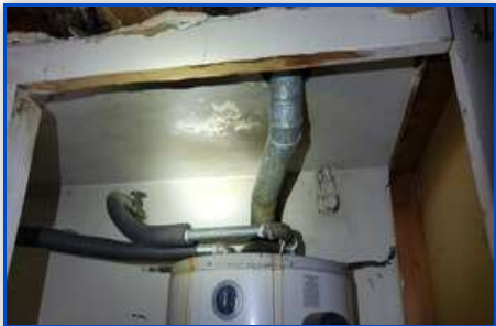
Location: 1745 WATER HEATER/GARAGE 2.1 Corroded galvanized water lines
