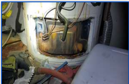
Location: 1745 WATER HEATER/GARAGE 5.1 Corrosion on tank
