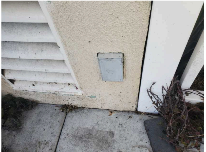
In-use cover not installed
