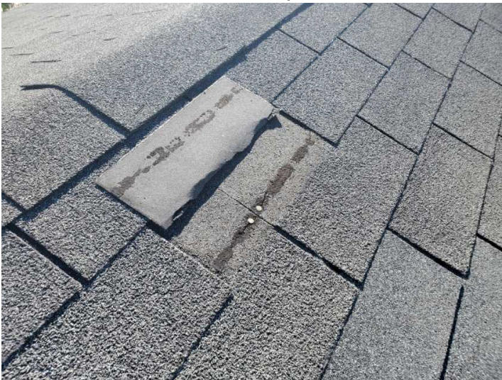
Damaged shingle
