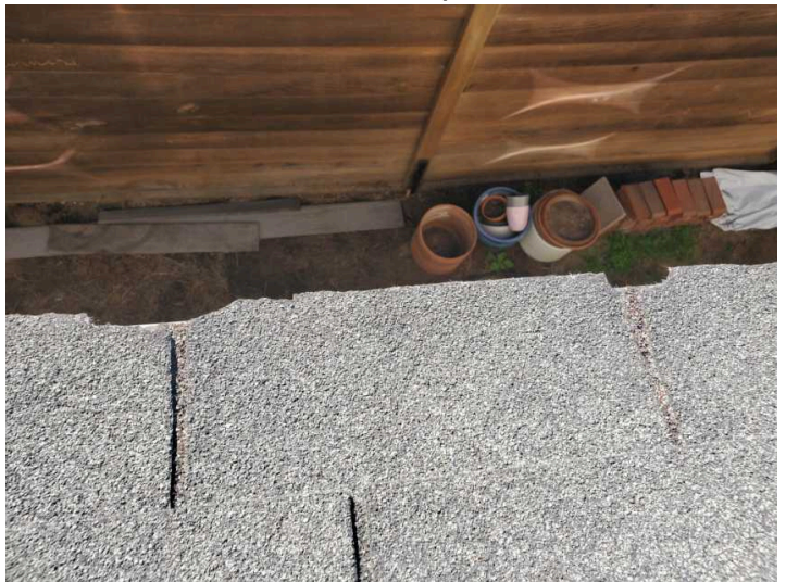
Damaged shingles
