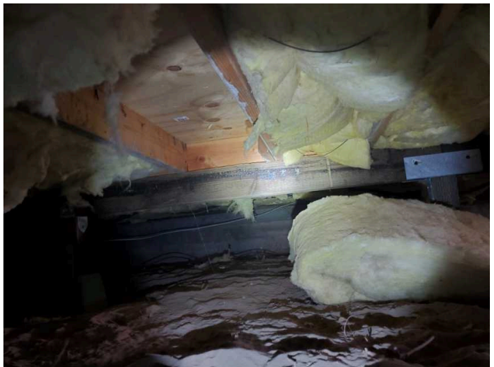
Insulation falling
