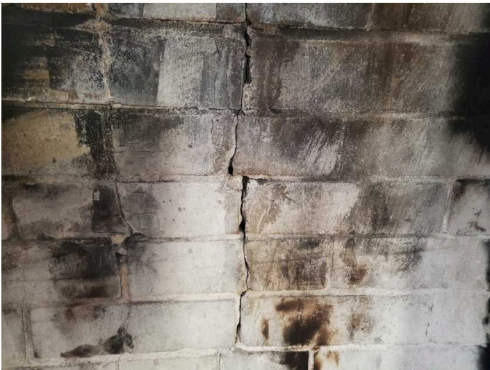
Damaged firebrick
