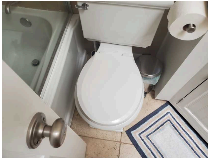
Improper clearance
