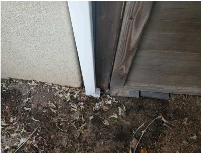
Downspout next to foundation
