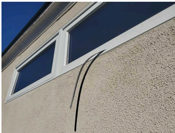
Weatherstripping damaged
