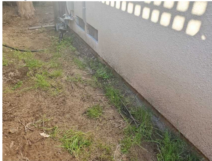
Poor grading
