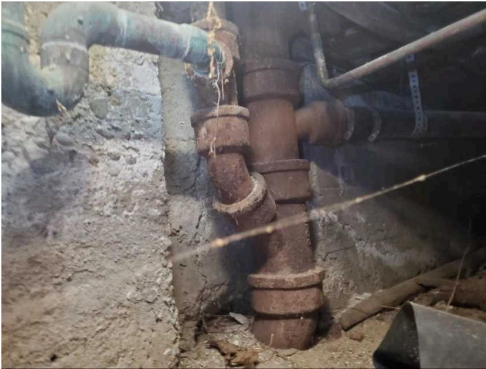
Original cast iron piping passing underground
