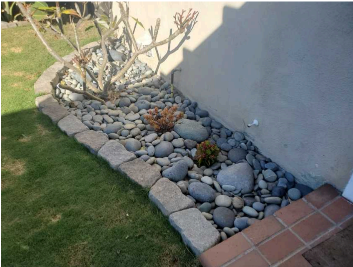
Poor grading
