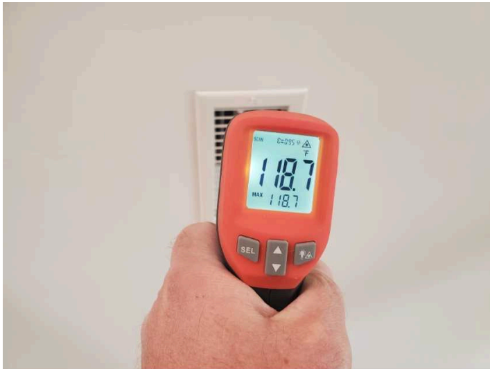
Heated temperature at register in back room
