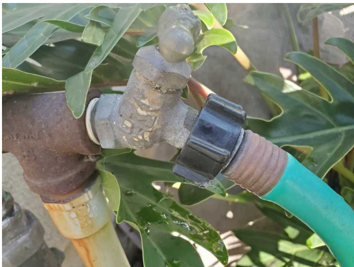
Missing anti-siphon valve
