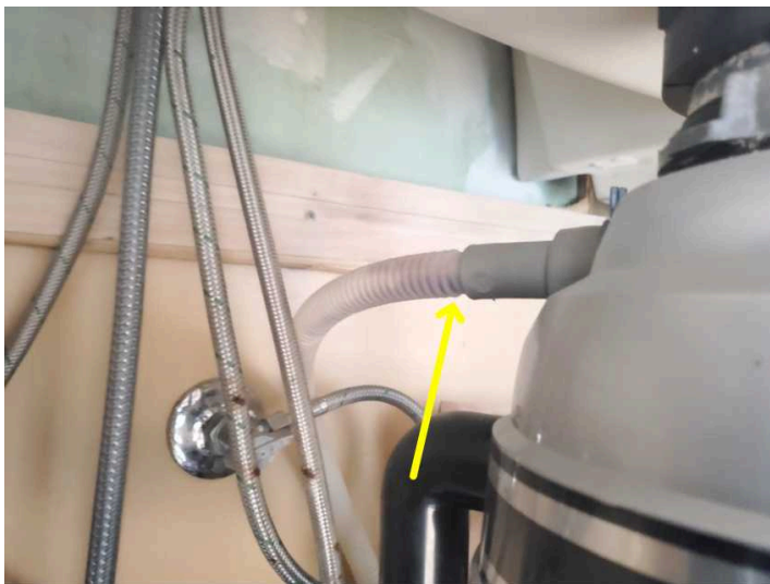
Improper drain connection
