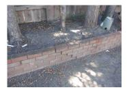
Vegetation is encroaching on the structure, and should be kept a minimum of twelve inches away for the general welfare of the walls and foundation.
